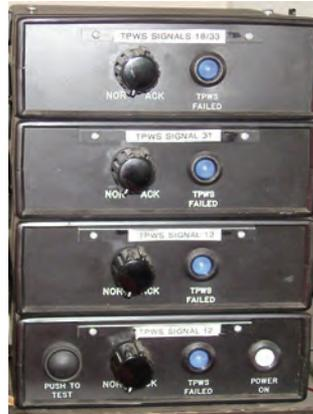
**Example of a failure indication unit**
